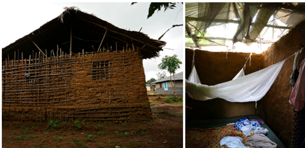
Fig. 3 Typical housing design in Bomi County, Liberia showing open gables and ceilings. Exterior photo shows the large gable allowing for cross-breeze and mosquito entry. Interior photo shows interior dividing walls extending approximately 2 m above the floor, an LLIN hung above the bed, and recycled LLINs sewn together to make a ceiling
