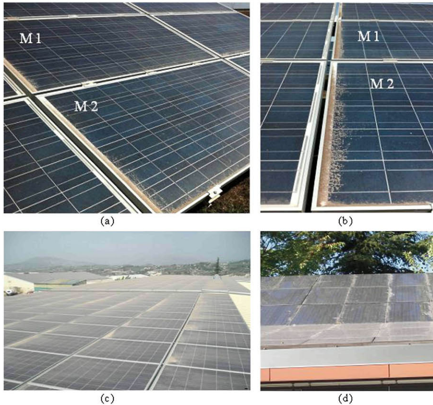
Figure 1. Non-uniform dust patterns spontaneously formed on PV modules and array surfaces. (a) At aforementioned Cartagena PV park, the dust shows a tendency to accumulate in the lower and on the left-hand part of several PV modules. (b) A detail of the previous figure shows that dust deposits do not only affect the free space between the solar cells and frames but also the solar cells' surface. (c) Dust on a close horizontal PV array on an industrial roof. (d) Dust on the roof of a so called "PV building".
