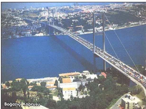
Figure 11. A general view of Istanbul Bogazici Bridge.
