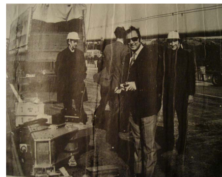
Figure 13. Shakers welded onto the deck by Skopje Institute.
