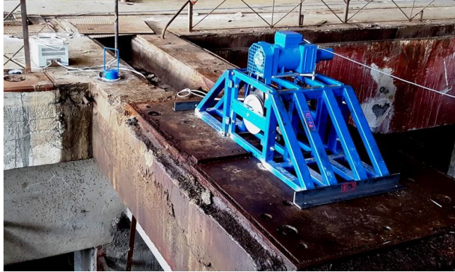
Fig. 4. Mechanical exciter at MB1 position on TGFS–6.
