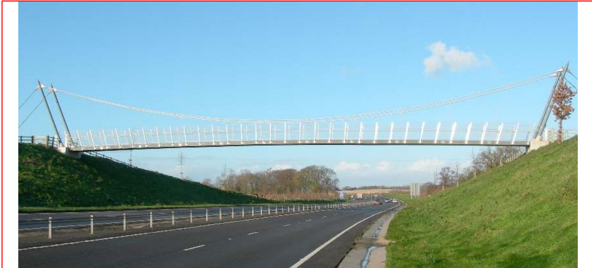
Fig. 1 An overview of the completed Wilcott footbridge.
