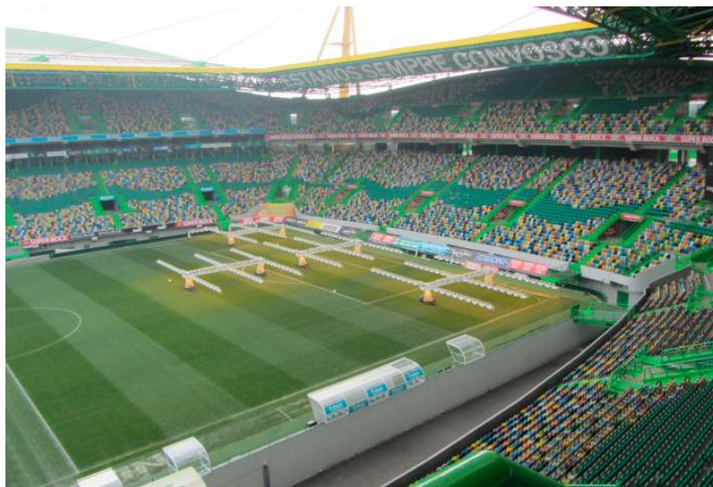
Figure 1. General view of the South grandstand.
