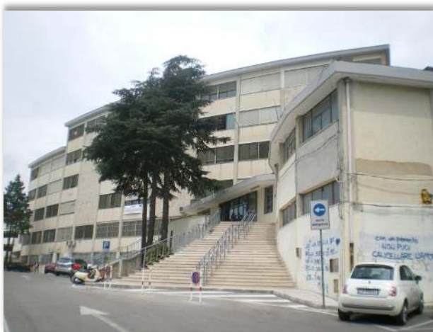
Figure 3. Building envelope of Liceo Classico E. Duni
