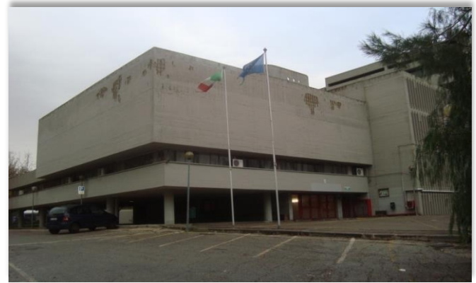
Figure 4. Building envelope of Liceo Scientifico D. Alighieri
