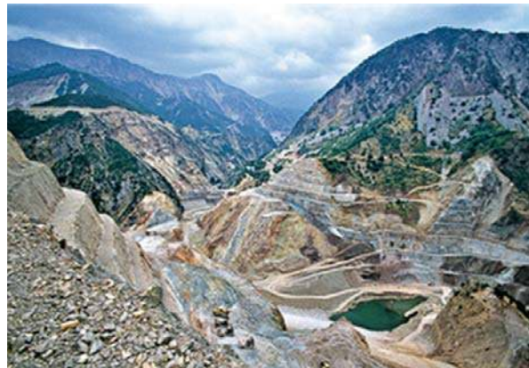
c: A view of Sykia dam.
