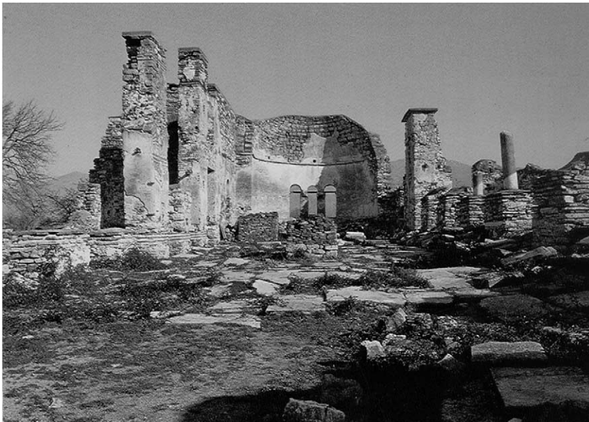
Fig. 7. The wall masonry of Aghios Achilleios basilica.
