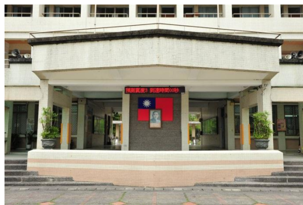
Figure 6. Character generator of the earthquake early warning system installed in Yilan Elementary School.
