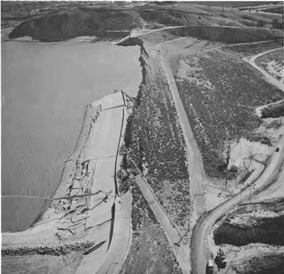
Fig. 1. View of Lower San Fernando Dam after Upstream Slope Slide in Earthquake of Feb. 9, 1971
