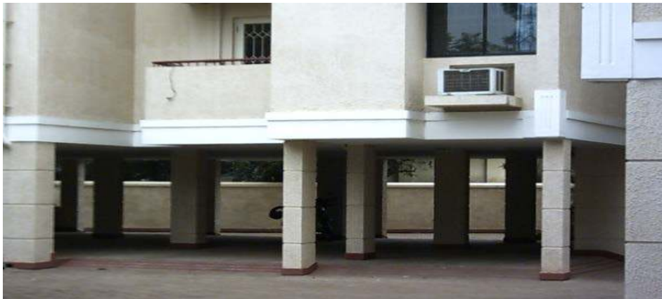
Fig. 1.1: Typical example of OGS building
