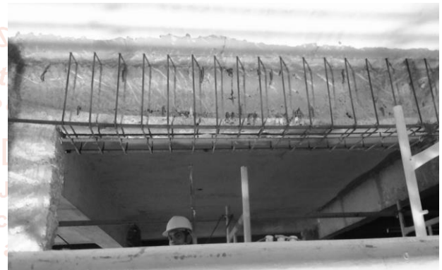
Fig. Beam Jacketing
