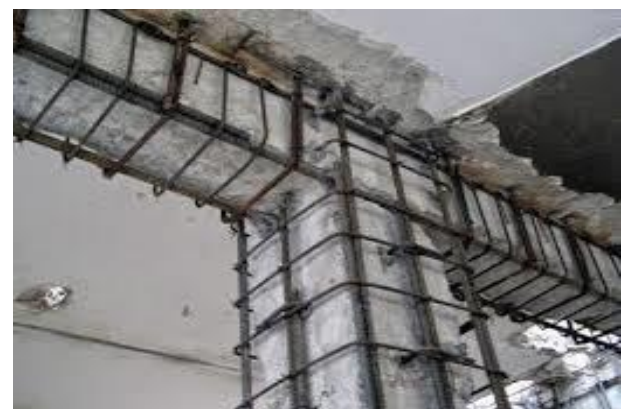
Fig. Beam column Jacketing
