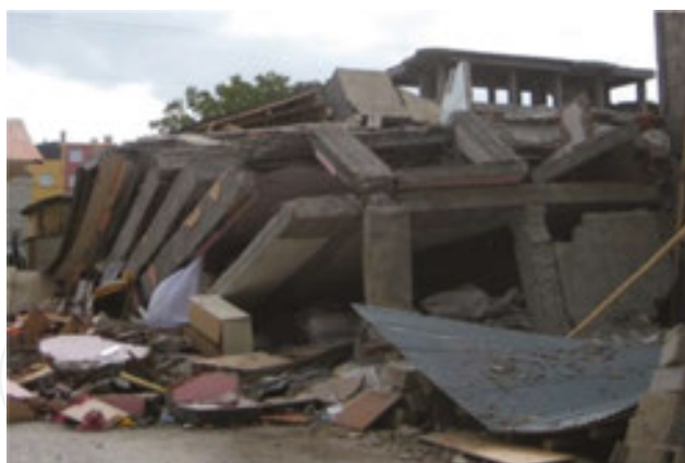
Figure 15. Failure of a building due to strong beam–weak column effect during the Van earthquake.
