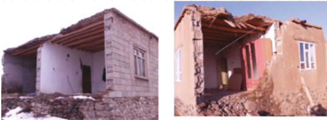
Figure 21. Out-of-plane mechanism of the brick buildings [42].
