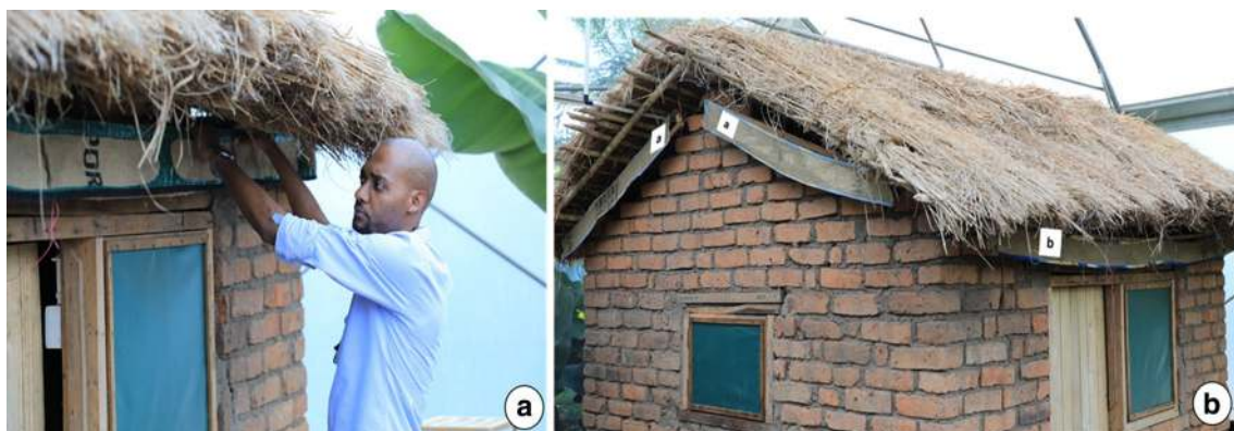
Fig. 2 Pictorial illustration of the eave ribbons and their installation along the eave-spaces of the experimental huts (a). In the current trials the eave ribbons were designed in lengths of either 1 m or 1.5 m, so multiple pieces were used to cover the entire eave space of the huts (b). However, the ribbons could be designed and manufactured with longer lengths, then cut to fit specific house sizes. The ribbons are fitted such that they do not completely cover the eave space, but also without directly touching the experimental hut surfaces, to avoid any contamination (b). During the tests, both the two experimental huts in the chamber were either fitted with or not fitted with the eave ribbons. At the end of each set of tests, the chambers were left free for at least 2 days and two nights to prevent residual effects of the treatments. Photographs by Emmanuel Mwanga
