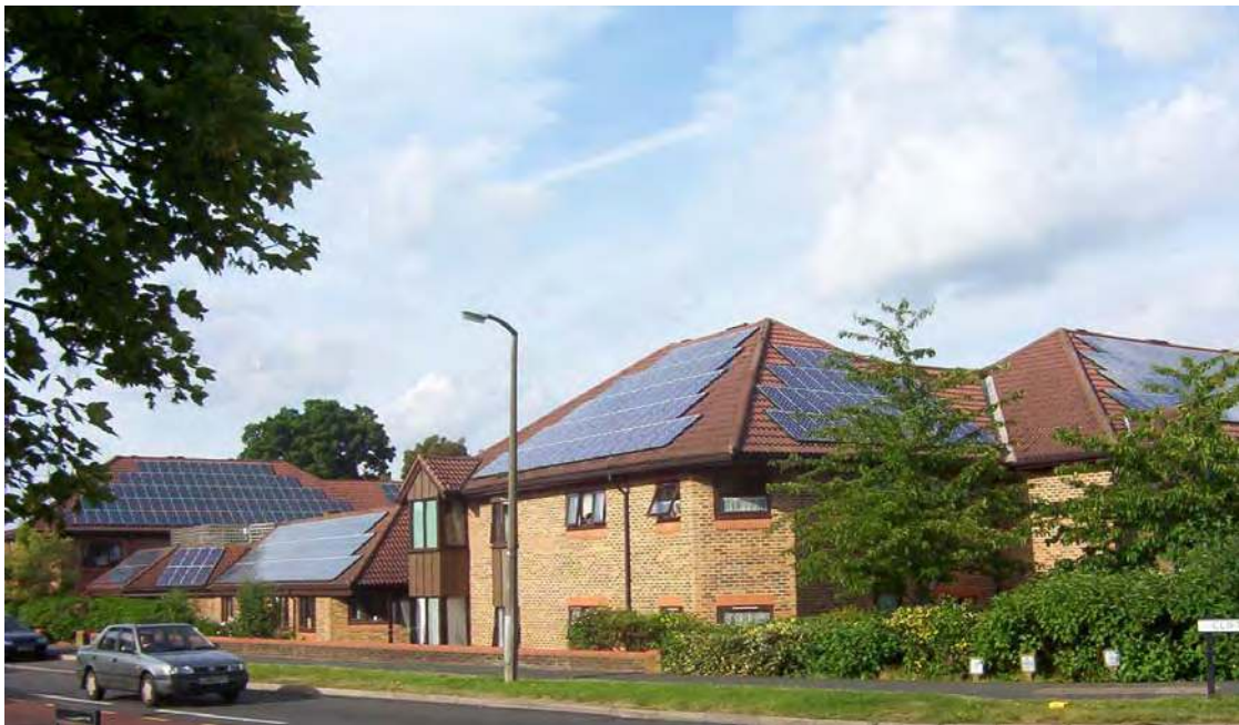
Plate 1: Photo voltaic cells on dwellings in Woking, England.
