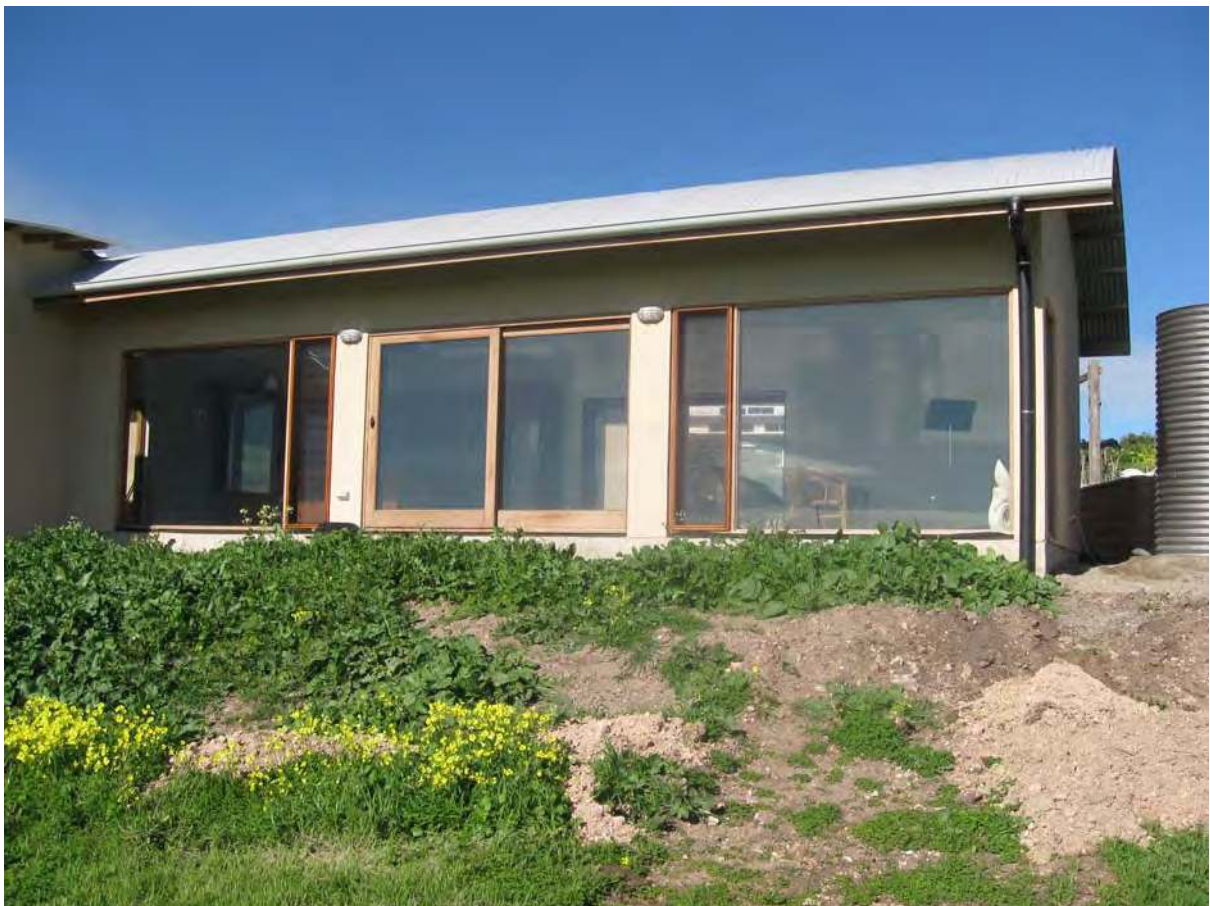
Plate 2: Passive Solar Orientation (at Aldinga Arts Eco Village)
