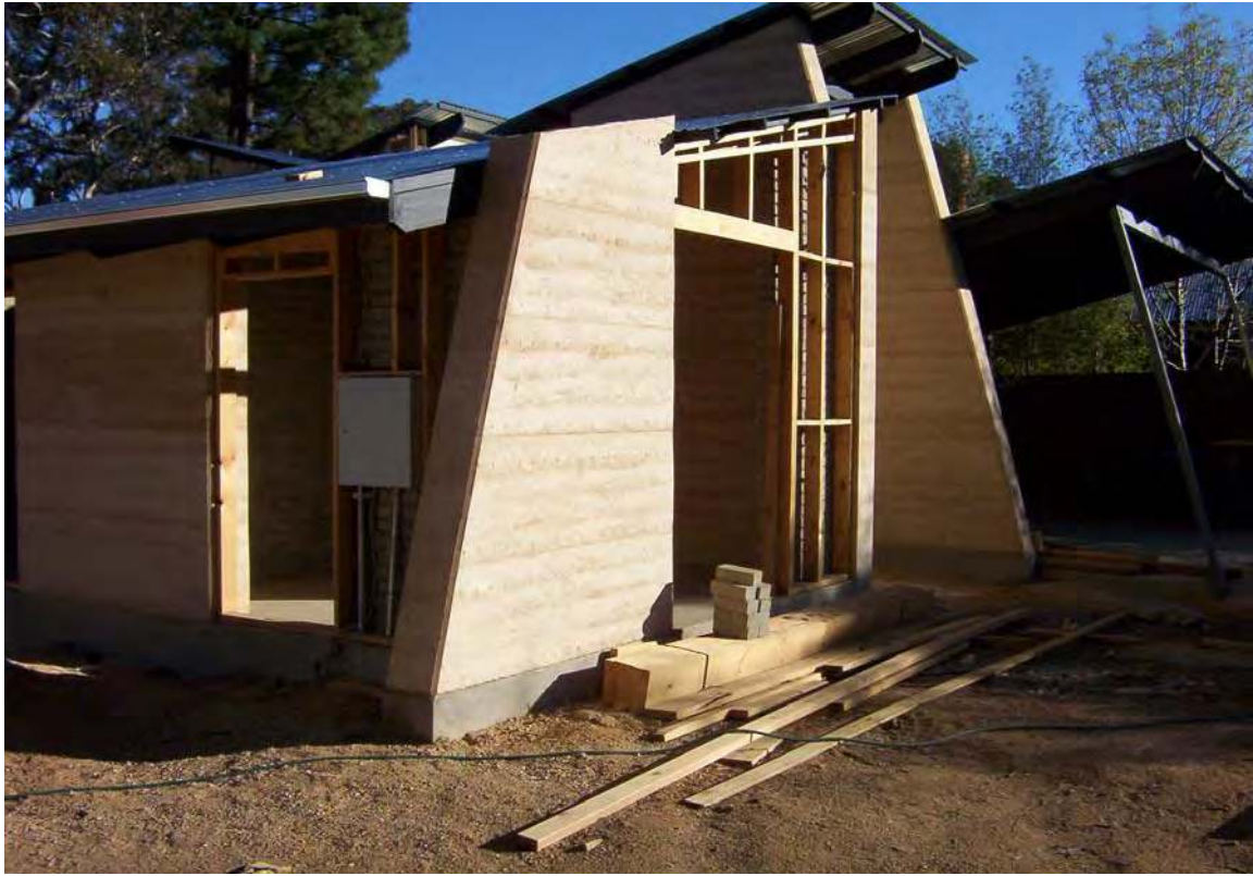
Plate 4: Rammed earth construction
