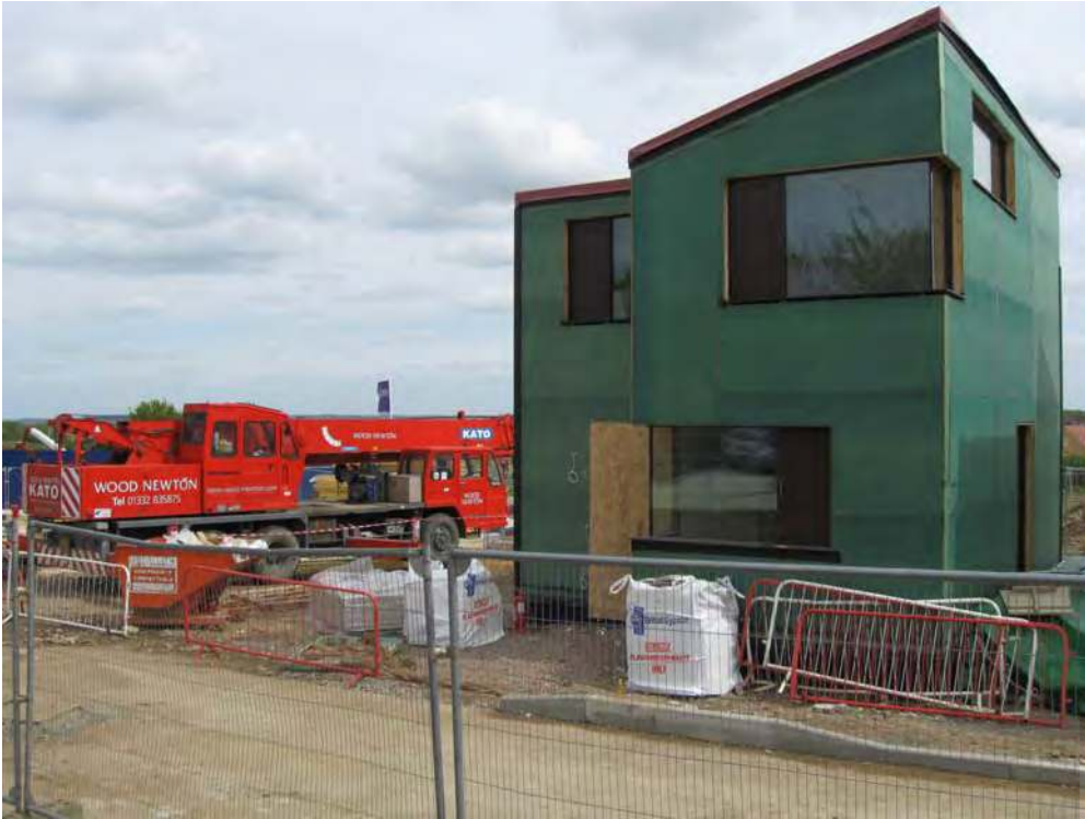
Plate 5: Prefabrication Construction Techniques (at Oxley Park, UK)
