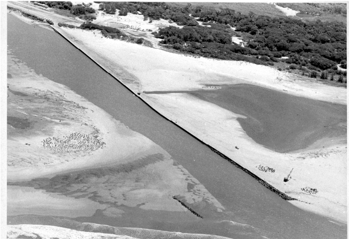
Fig. 7. Aerial photograph of the St Lucia mouth showing the partially constructed groynes designed to stabilize the north and south banks of the estuary. In the mid-left of the picture is a stockpile of dolosse used to reinforce the groynes adjacent to the sea (Photo: R.H. Taylor, 1976).
