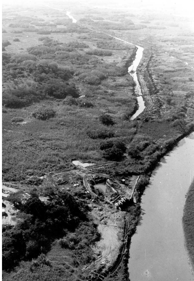
Fig. 8. Aerial photograph showing the partially constructed intake works on the bank of the Mfolozi River in the foreground, with the Link Canal to the St Lucia Estuary under excavation in the background (Photo: R.H. Taylor, 1983).
