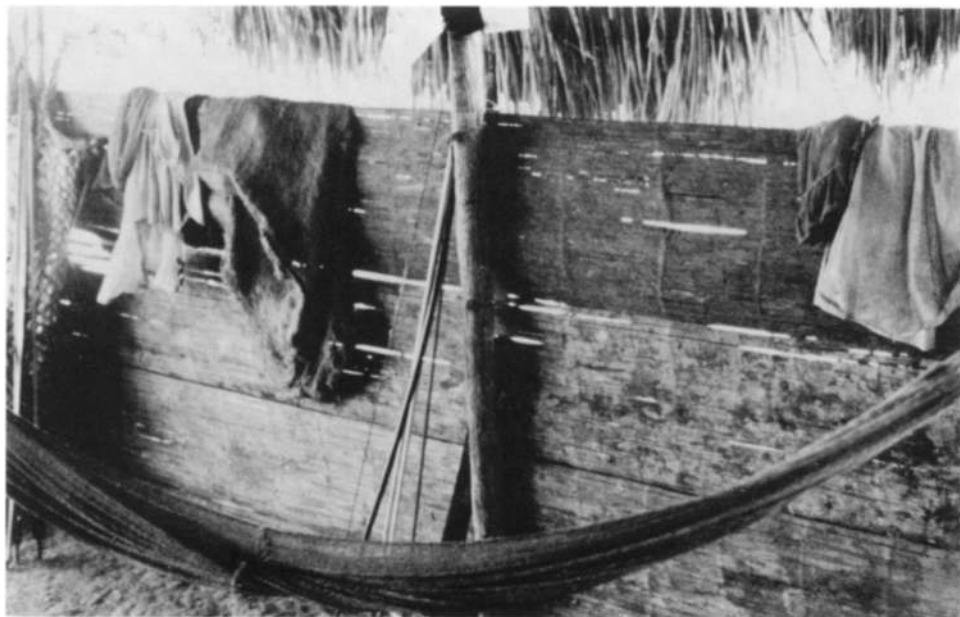
Fig. 10. The interior of a Guahibo dwelling. Note the hammock of Astrocaryum chambira fiber, the wall of an unrolled trunk of Socratea exorrhiza , and the hunting bow carved from ataíto , the wood of Jessenia bataua .
