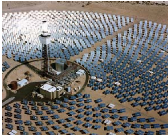
Figure A-6 10 MW Solar Two Power Tower System (Source: NREL)
