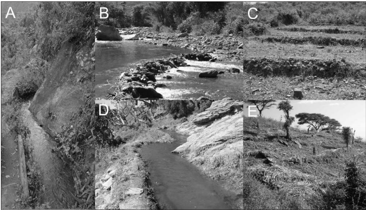
Figure 2: A. Stone lined irrigation canal, Pokot. B. Dam and intake canal, Pokot. C. Stone terracing, Pokot. D. Irrigation canal, Marakwet. E. Simple 'trash' terracing, Marakwet.
