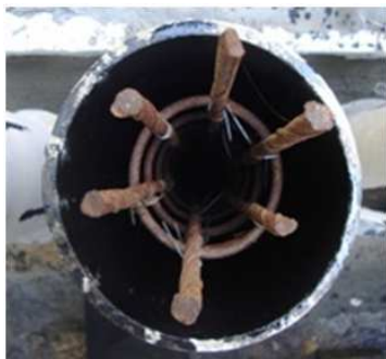
Fig. 1: Reinforcement cage in formwork
