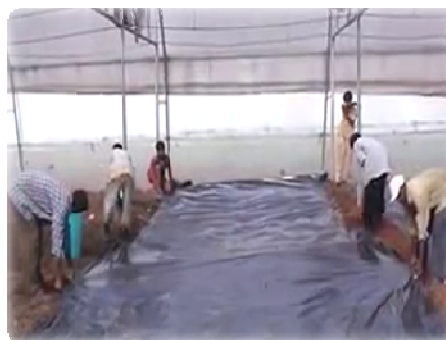
Fig: 2b. Polyethylene Sheet Covering
