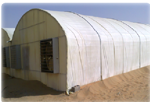
Fig: 1a. Side View of Greenhouse
