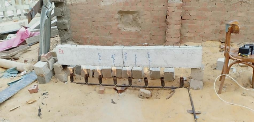
Fig. 19: During the fire for the beam (F-B).
