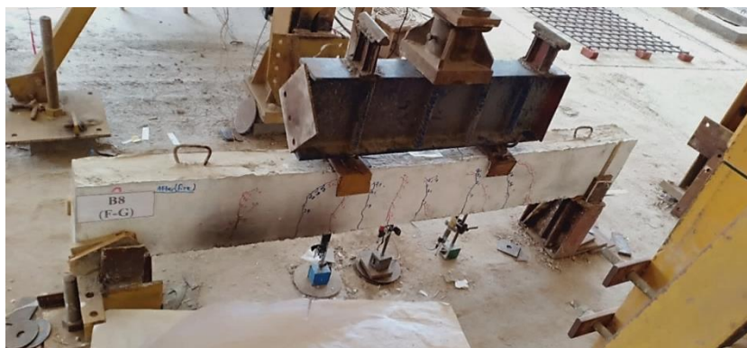
Fig. 26: After the fire and loading at failure load for the beam (F-G).
