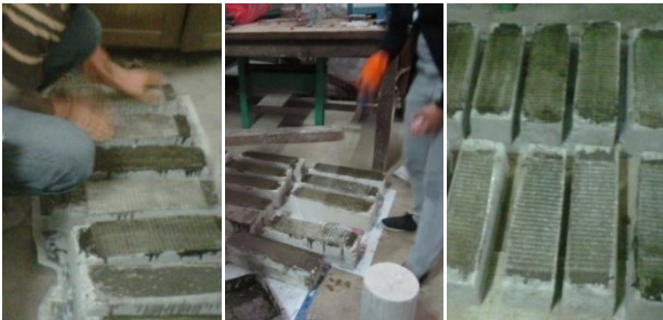
Fig. 3. Installation of GFRP sheet on the beam.
