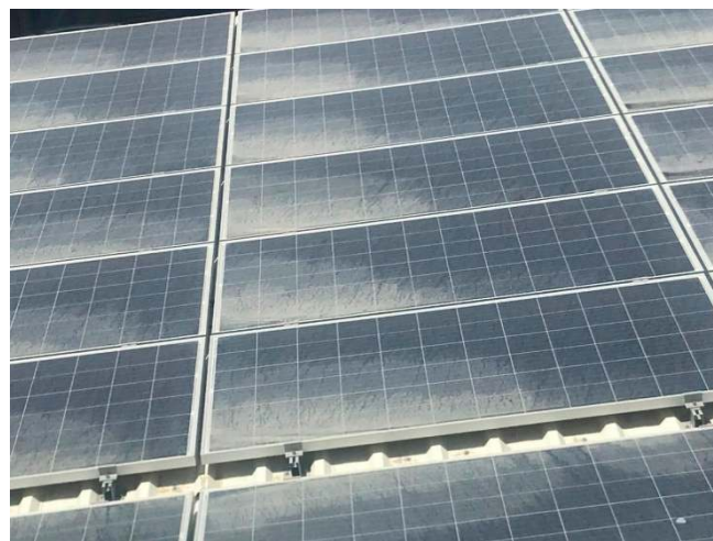
Figure 9. Photograph of partial section of the modules showing the high dust accumulation.
