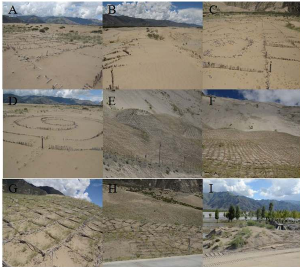
Figure 6. Status of revegetation in the middle reaches of Yarlung Zangbo River Basin in July 2016. (A–D) are the sand barrier of straw by local residents and government; (E–H) are the grass checkerboard barriers by local residents and government; I is populus and u. pumila plantation planted by local forestry bureau.
