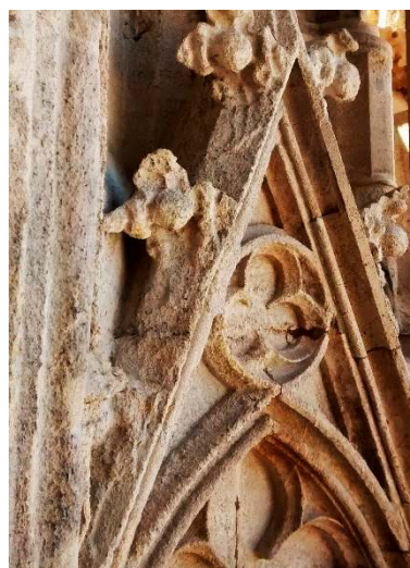
Figure 1. An outdoor decorated frame of Auer limestone of St. Stephen's Cathedral façade in Vienna (Austria), showing extensive erosion and loss of detail after exposure to weathering agents.
