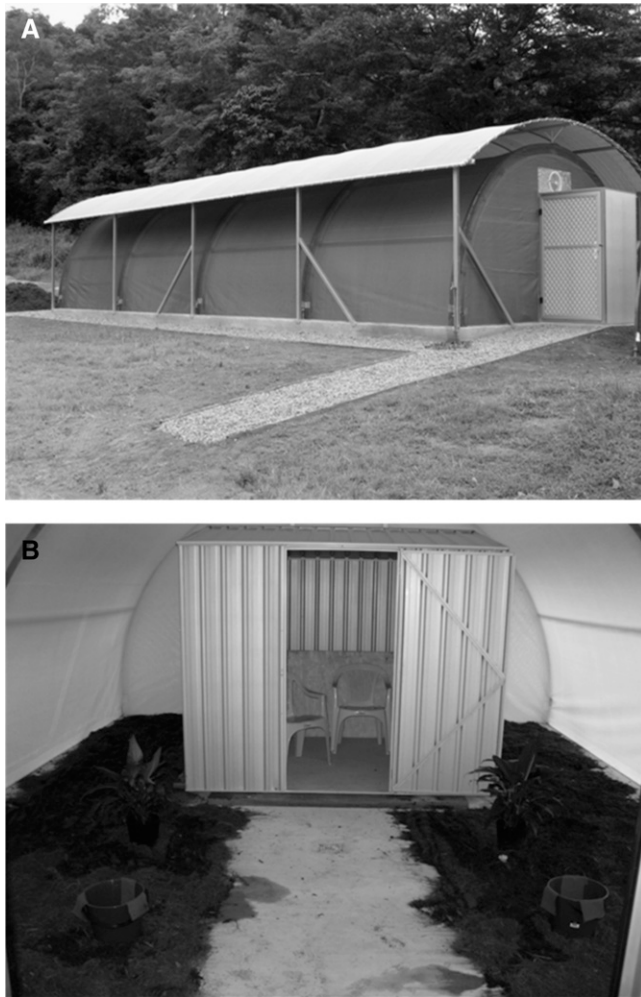
FIGURE 2. Semi-field cage at James Cook University, Smithfield Campus, Cairns, Queensland, Australia. A , Structure contains two cages bisected by a transverse double-walled partition made of Tentex screening. Cage B is to the north (left in the photograph) and cage A is to the south (right in the photograph). B , Interior shed simulating a human-inhabited structure.
