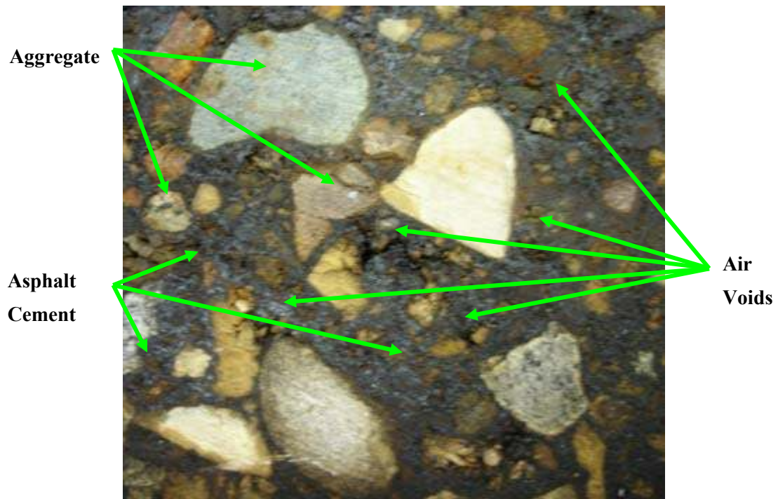
Figure 2.11 Saw-Cut Asphalt Concrete Surface
