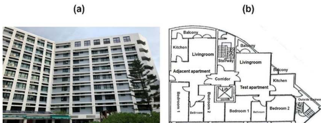
Figure 1. (a) The multistory apartment building; (b) floor layout; identical on each floor.
