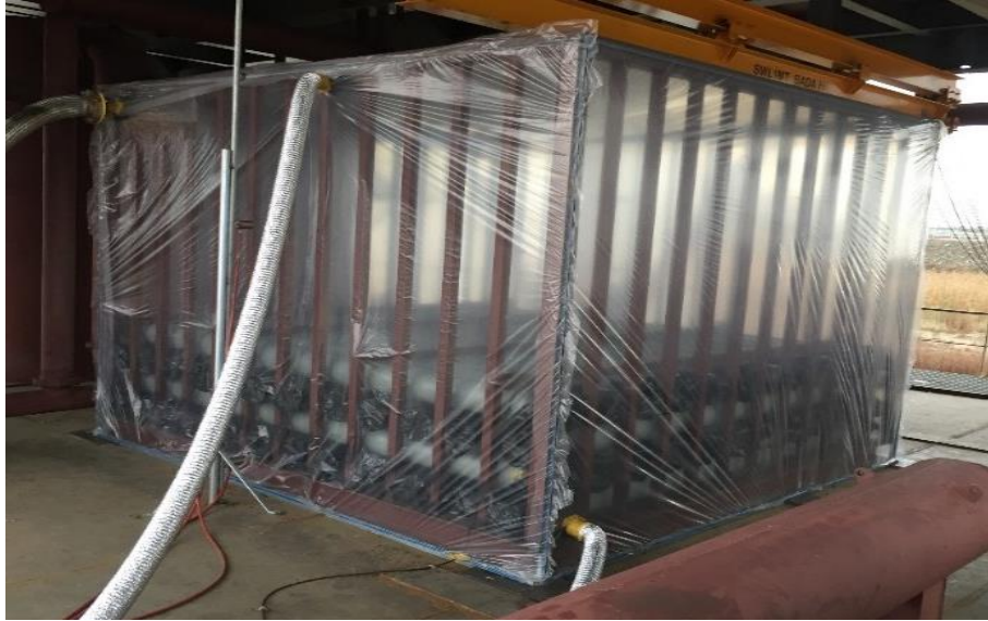
Figure 5 Pipe rack structure covered by a very thin plastic sheet
