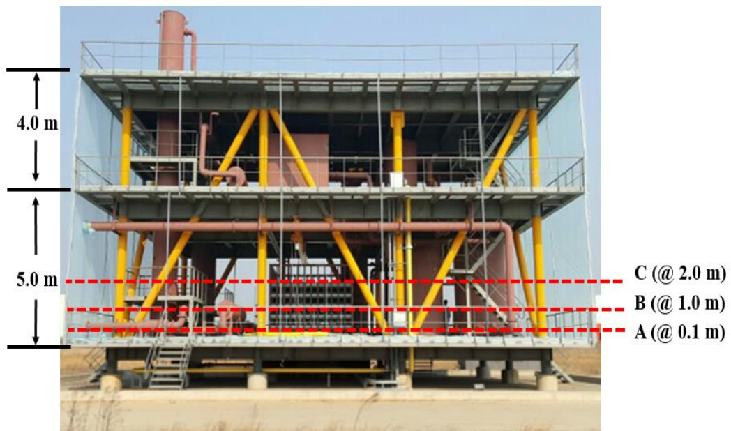
(a) Elevation view of pressure sensors
