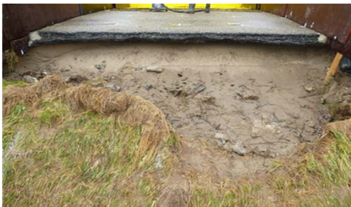
Figure 3.7 Inspection road on the crest of the dike
