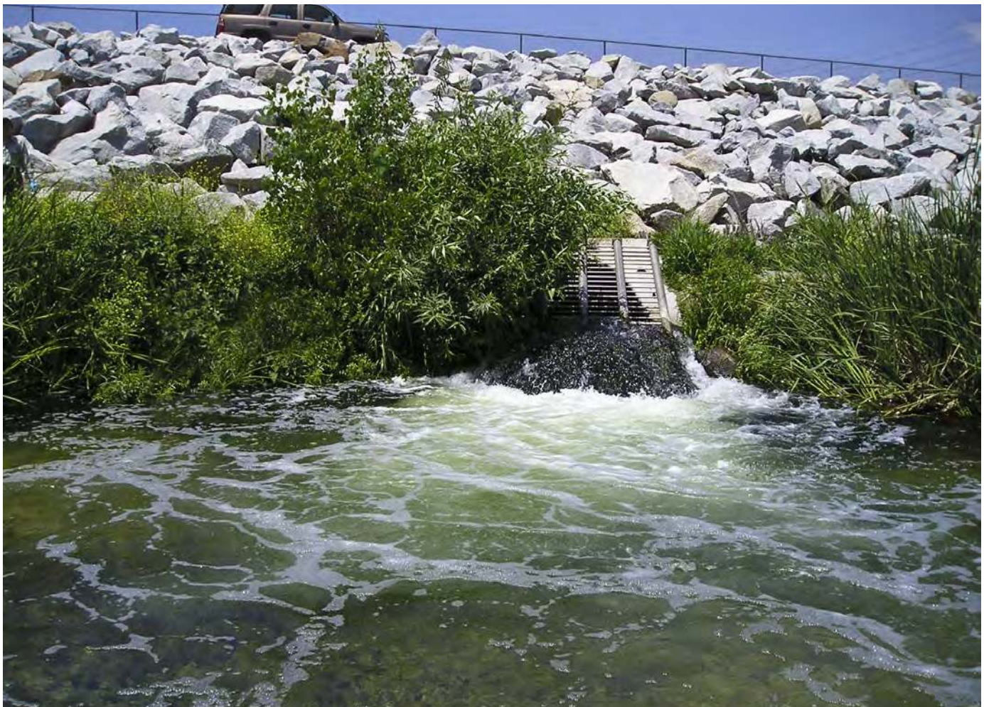
Figure 3. Plunge pool below a discharge site for tertiary treated wastewater effluent, Colton, Calif. Photograph by Judy Gibson.
