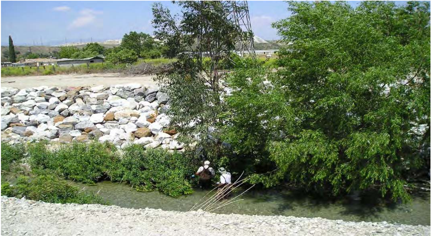
Figure 4. Rialto Drain below West Agua Mansa Road, Colton, Calif.
