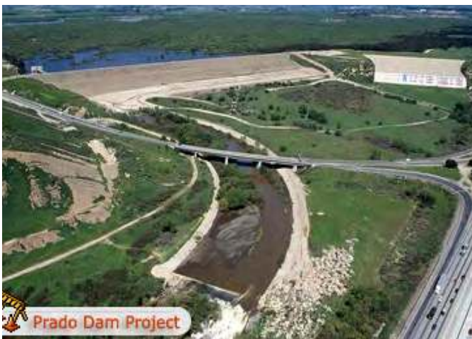
Figure 5. Sediment control structure below Prado Dam, near Corona, Calif.
