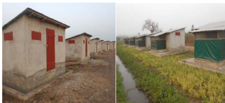
Fig. 1 Experimental hut station at Covè, Benin
