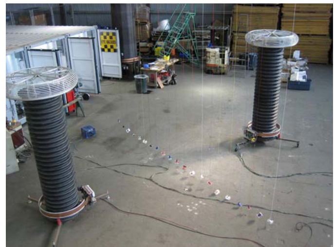
Fig. 5. Electrostatic test curtain in position between transformers.
