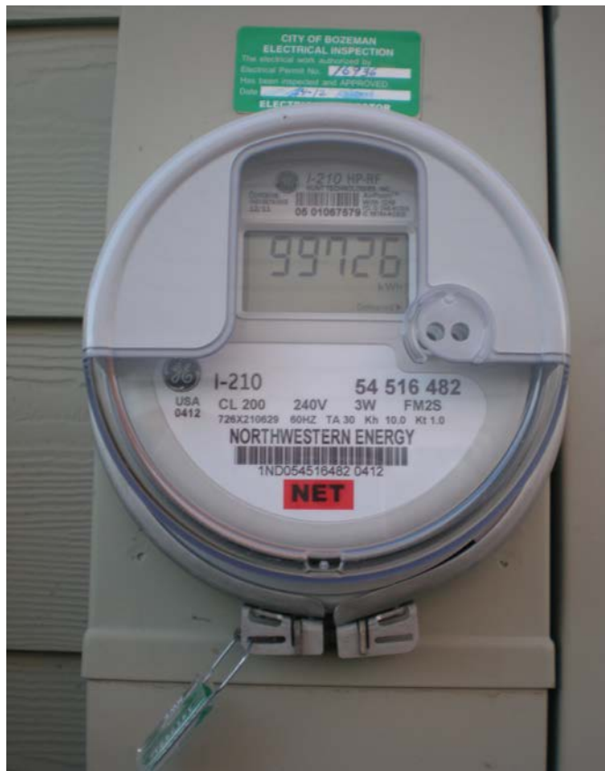
Fig. 1. A smart meter at a residence. Photo sourced from National Renewable Energy Laboratory (NREL) database, PIX 21394.
