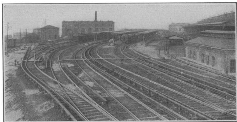
FIG. 9.—View of electrified yard at Camden terminal
