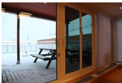
Fig. 7. Part of an office equipped with electrochromic glazing, with one window in its transparent state and two windows in their dark state.
