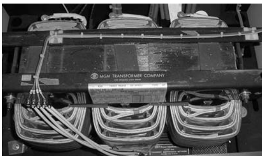
Figure 4-3: Open winding structure with air channels to enhance convective cooling
