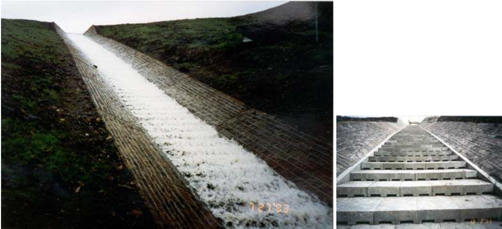
(B) Brushes Clough dam (UK) in 1993 (Courtesy of Mr Gardiner, NWW) - Left: small overflow; Right: details of the concrete block placement
