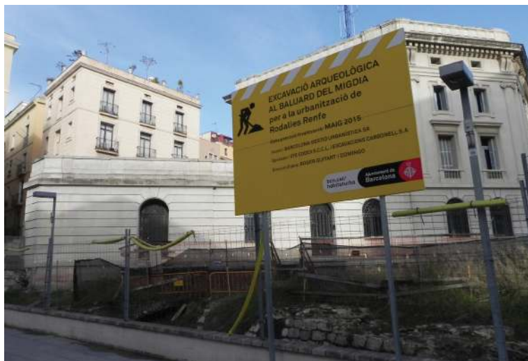
Figure 14. Works on the Bastion of Noon placed on the frontier between the neighbors of Barceloneta and La Ribera during 2014-2015. Ana Pastor.
