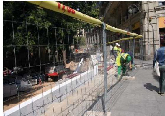
Figure 13. Laborers working on the construction of a “podium” to enhance the Roman Walls of Barcelona, street Tapineria, on May 2016. Ana Pastor.
