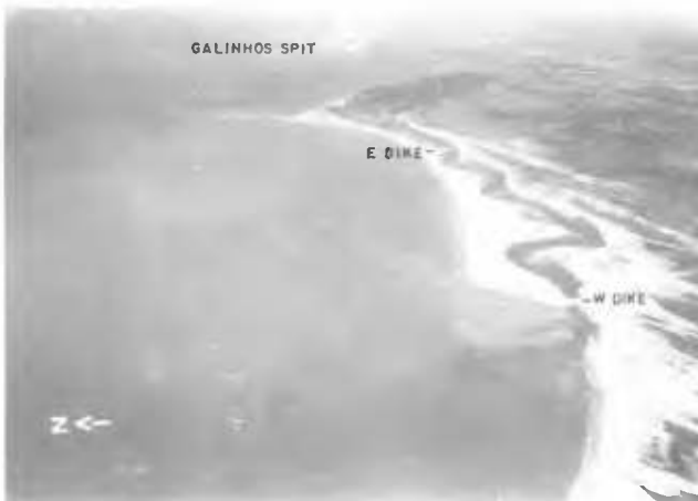
Figure 12. West Dike (13 Days After Closure) Date: 04/07/88 Hour: 14:27 W.L. = +0.8m
