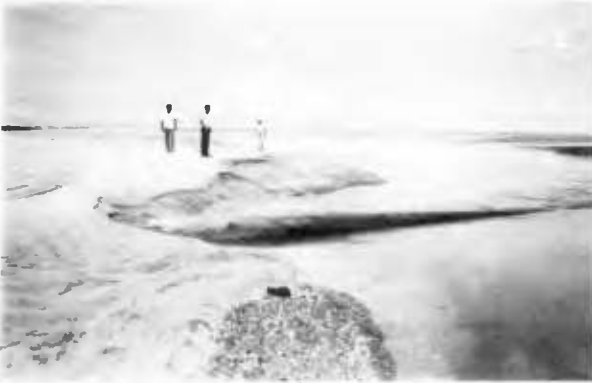
Figure 7. Gas Pipeline Date: 03/02/88 Hour: 09:08 W.L.= +0.9m (ebb tide)
