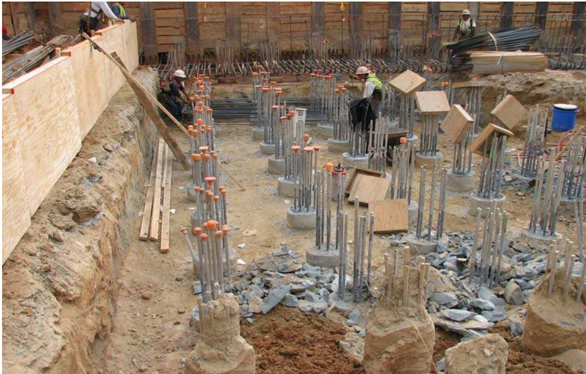
Figure 38-Picture of ACIP pile butt's and steel reinforcement for large mat foundation.
