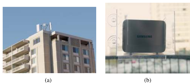
FIGURE 8. (a) Verizon 5G infrastructure (smallcell) on roof, and (b) Samsung home unit (femtocell) attached on window [42].
