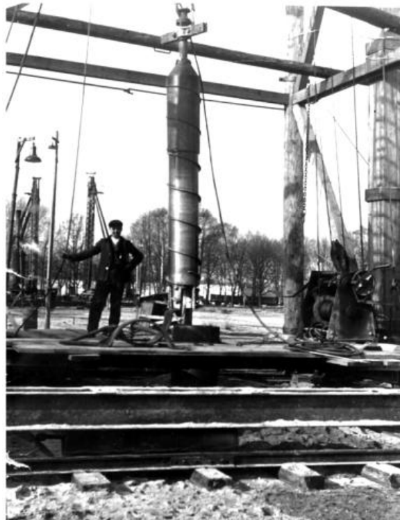
Figure 7-4. A 1937 photograph of an early vibrocompaction system or “Pfeilerruetzler” (vibrating pile). (Photograph by W.L. Degen, courtesy of W.S. Degen, Vibro Systems Inc.).
