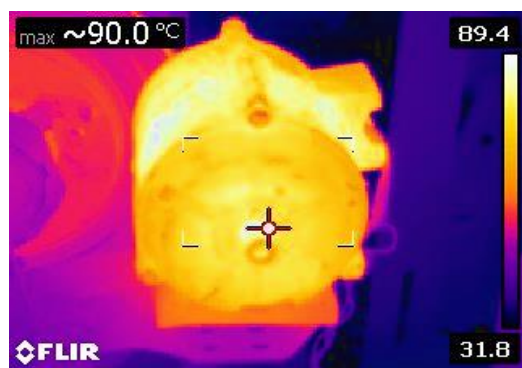
FIGURE 16. Infrared Thermography of Motor with Filter configuration
