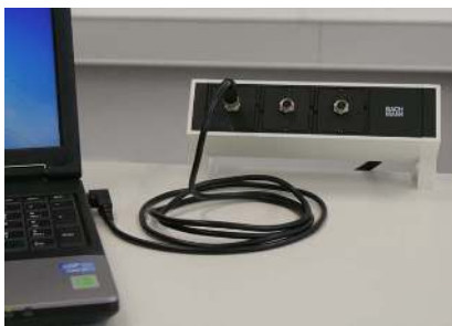
Fig. 7. Frame connector with three output sockets of the 24 VDC nano grid
