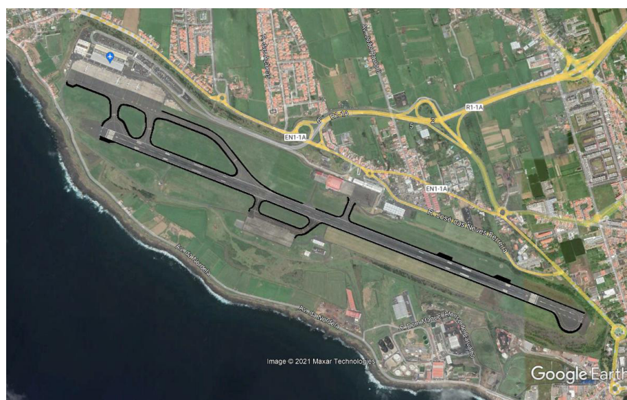
Figure 2. Installation aerial view overlaid with implementation zone.
