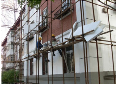
Figure 4. Two Workers Install Insulation in a Typical Chinese Residential Building
