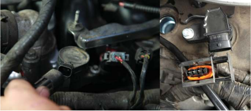
Fig. 2. The supply to the ignition coil pack was disconnected in order to induce a complete misfire on individual cylinders.
